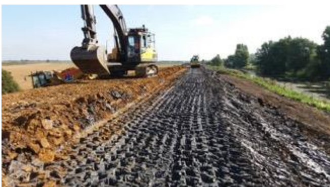
Constructing the clay layer on the SLBB at Sutton Gault
